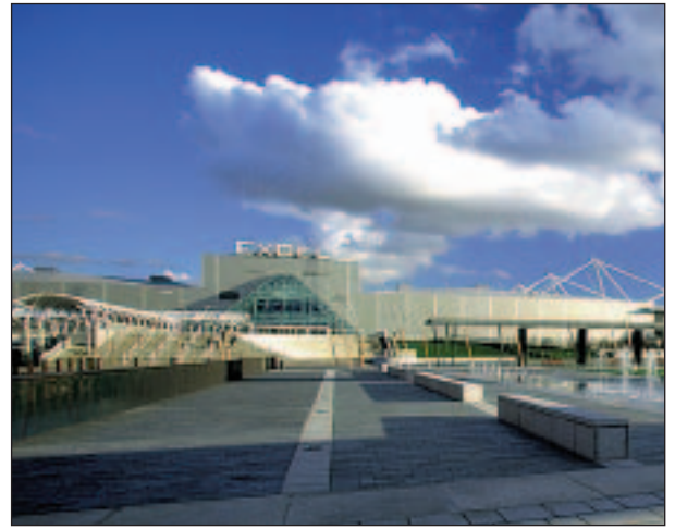
The New ExCel Pavilion
