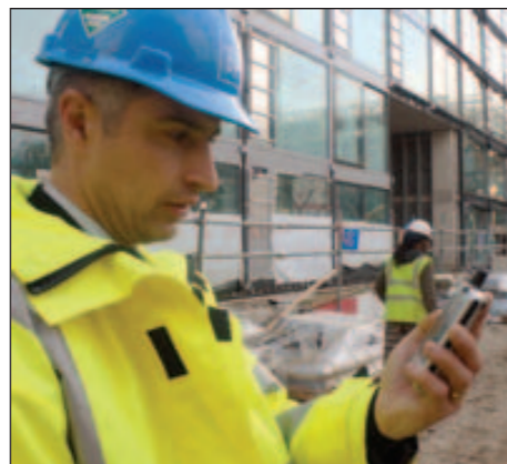
Testing, testing - SAV's Ian Stripp checks the remote reading facility for the energy meters at Highbury Corner.
